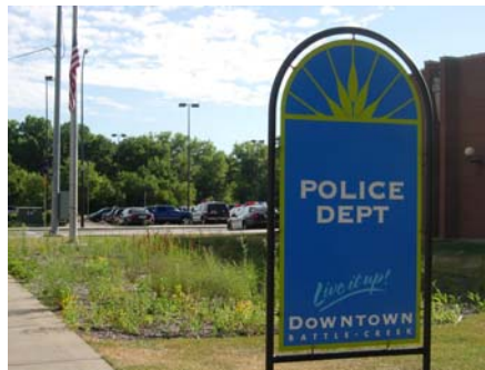
Rain garden in front of the Battle Creek Police Department building.
