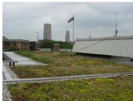
Vegetated roof on the Battle Creek Police Department building.
